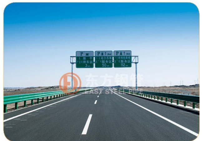
Beijing-Urumqi Expressway Project
